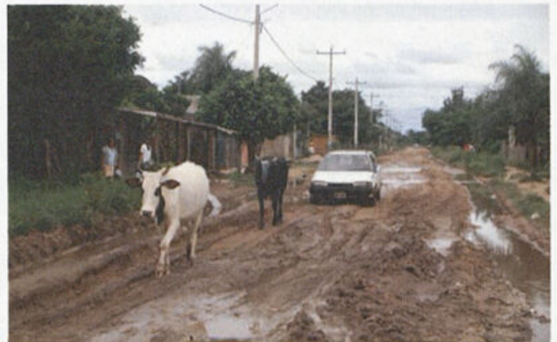
Plan 3000 has both rural and urban characteristics, with infrastructure and other basic services largely absent. Photo by David Bluestone.
