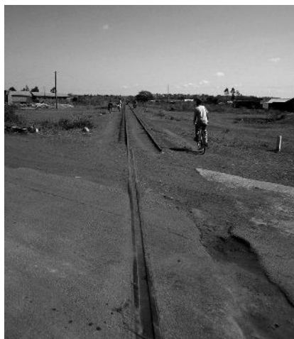
Caption: A photograph taken by the author shows deteriorating meter-gauge rail in Uganda likely laid by the
