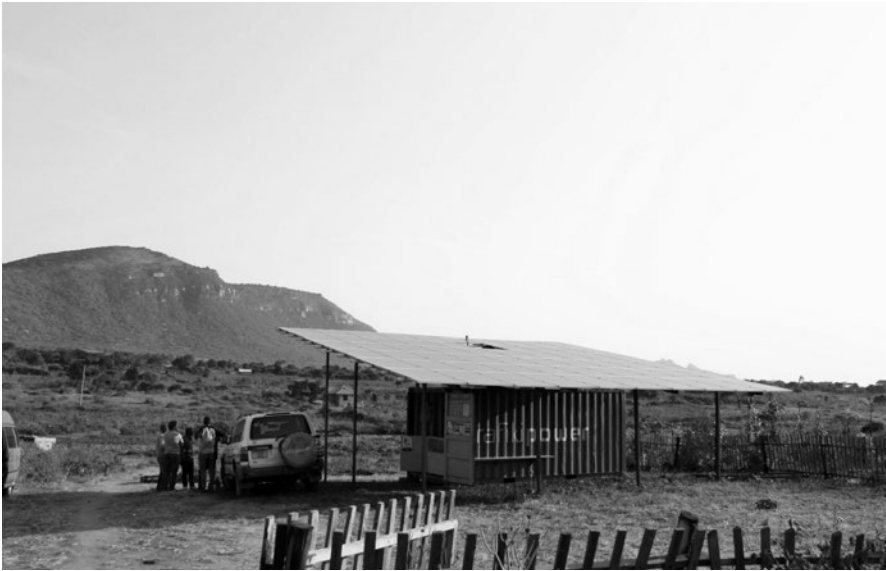
Figure 1: Mini-grid site in East Africa providing power to over 200 rural homes and businesses
